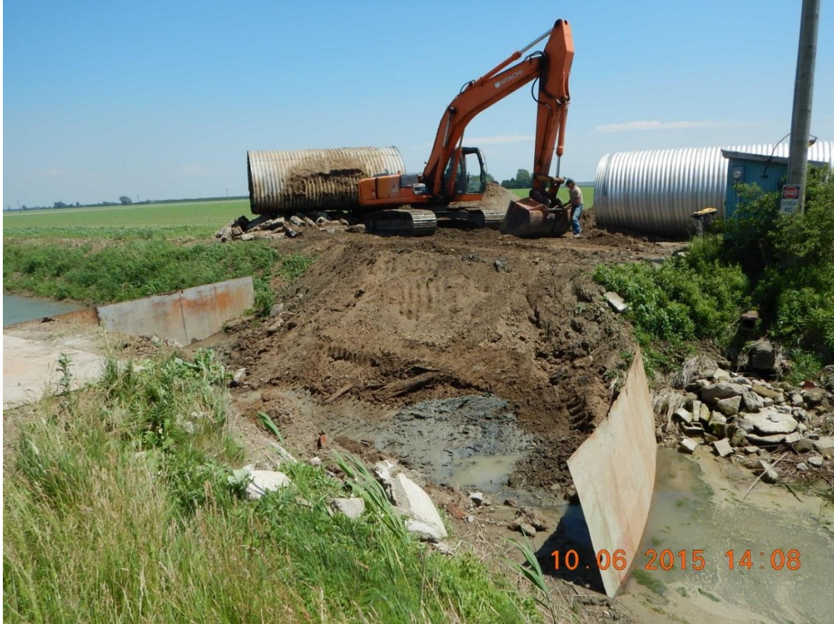
Figure 2. Isolation of Site
