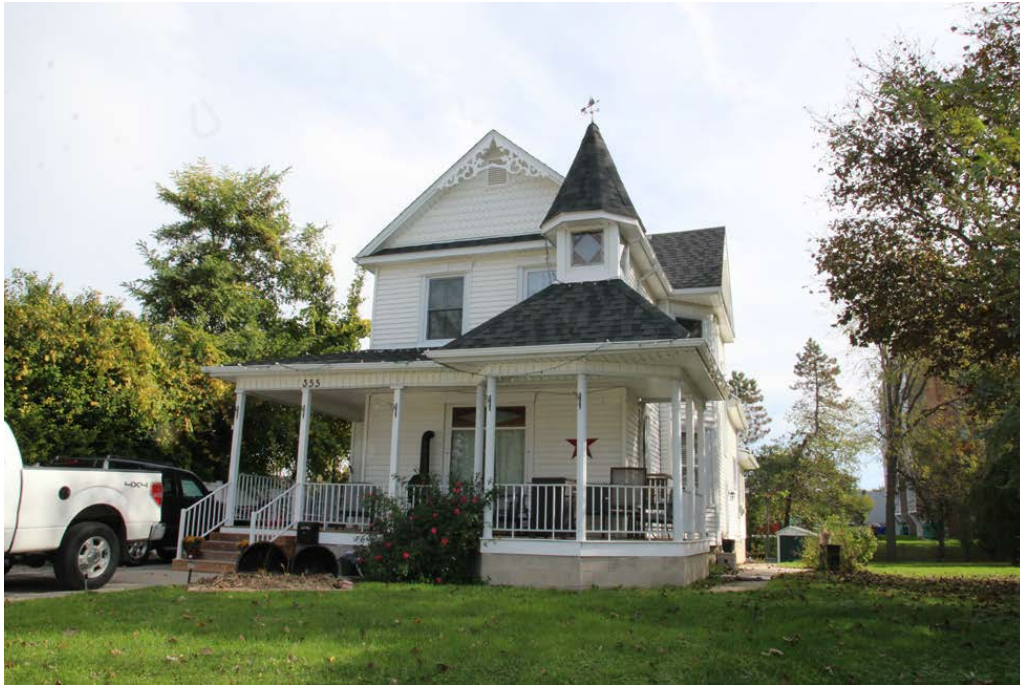
West Façade; October 2021
