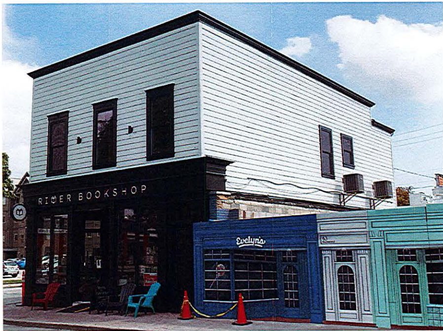
West façade and main facades of the Thomas Drug Store (August 27, 2021)
