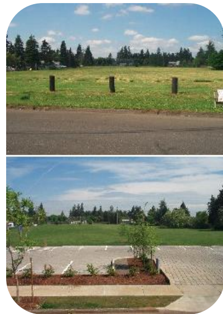
Figure 2: Before (above) and after (below) East Holladay Park porous parking lot construction (City of Portland, 2007)
