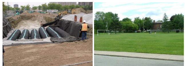
Figure 1: During and after construction (City of Toronto, 2009)
