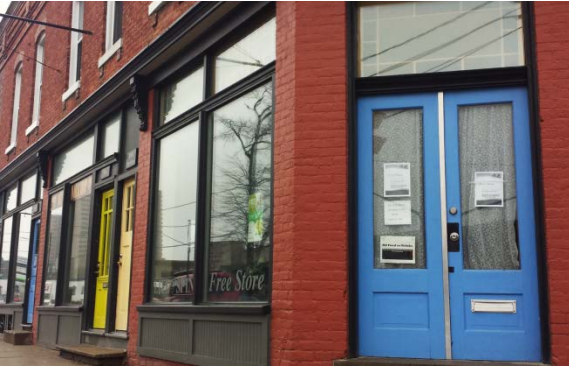
Transom windows above the display windows and doors
