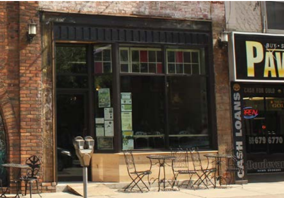
Wood base panel across bottom of display windows
