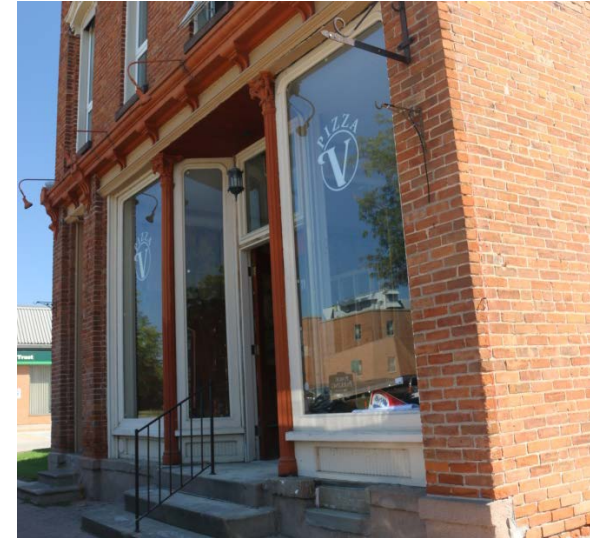
Recessed Entryway, lit with sconce and gooseneck lights and large transparent glass door and windows
