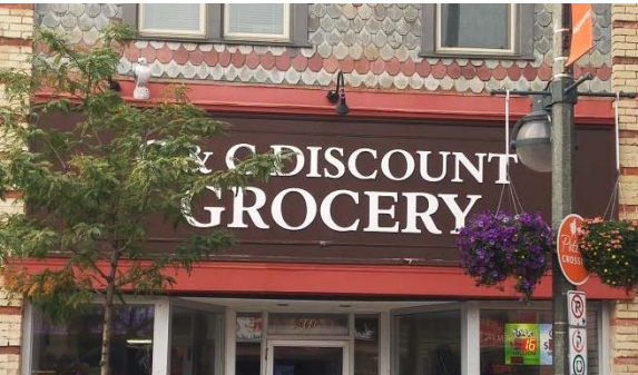
Fascia sign using raised lettering on a sign board.
