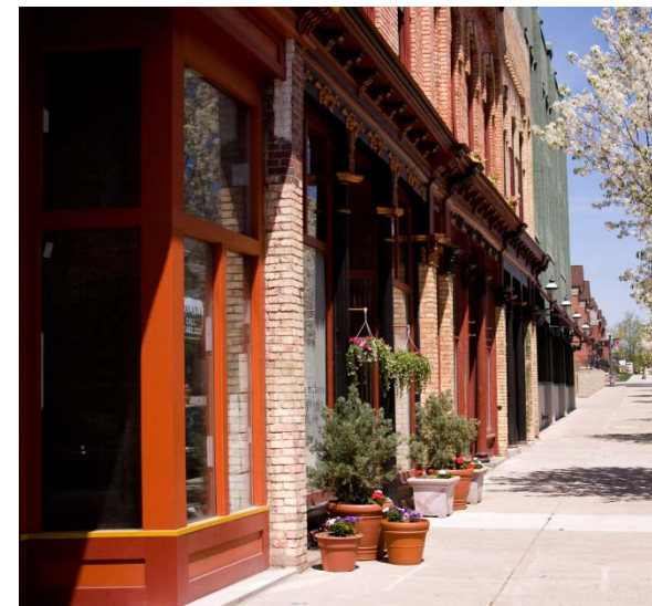
Cornices at the top of the ground floor and pilasters dividing bays for each storefront
