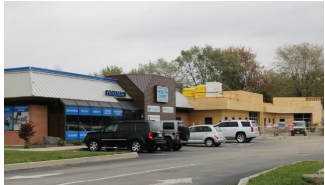
New medical office under construction, Sandwich Street
