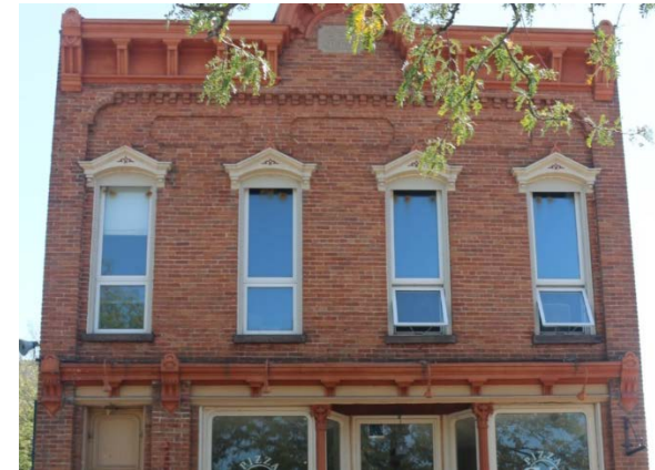
Existing windows with decorative lintel above and raised brick quoins along the building edges
