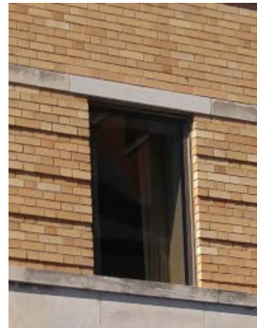
Modern yellow brick façade with grey concrete accents
