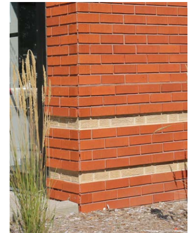
Modern red brick façade with yellow brick accents
