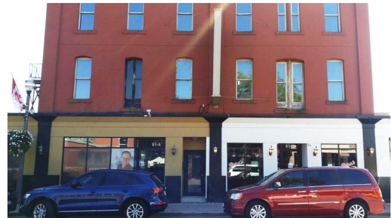
Windows and pillars create vertical divisions along the façade and cornices and windows divide up the height of the building
