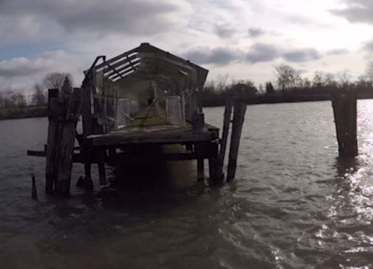
Figure 2-2 View of Northern end of pier looking along bent line 14 toward the South-East.
