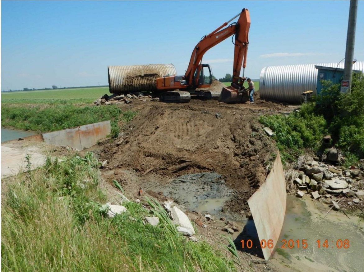
Figure 2. Isolation of Site
