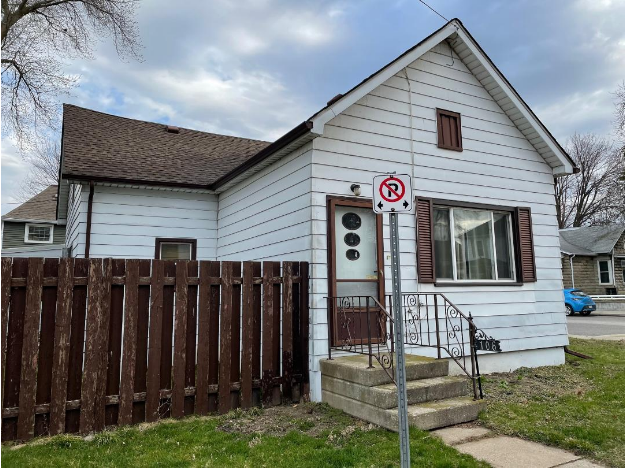
South Façade, Apr. 11, 2022
