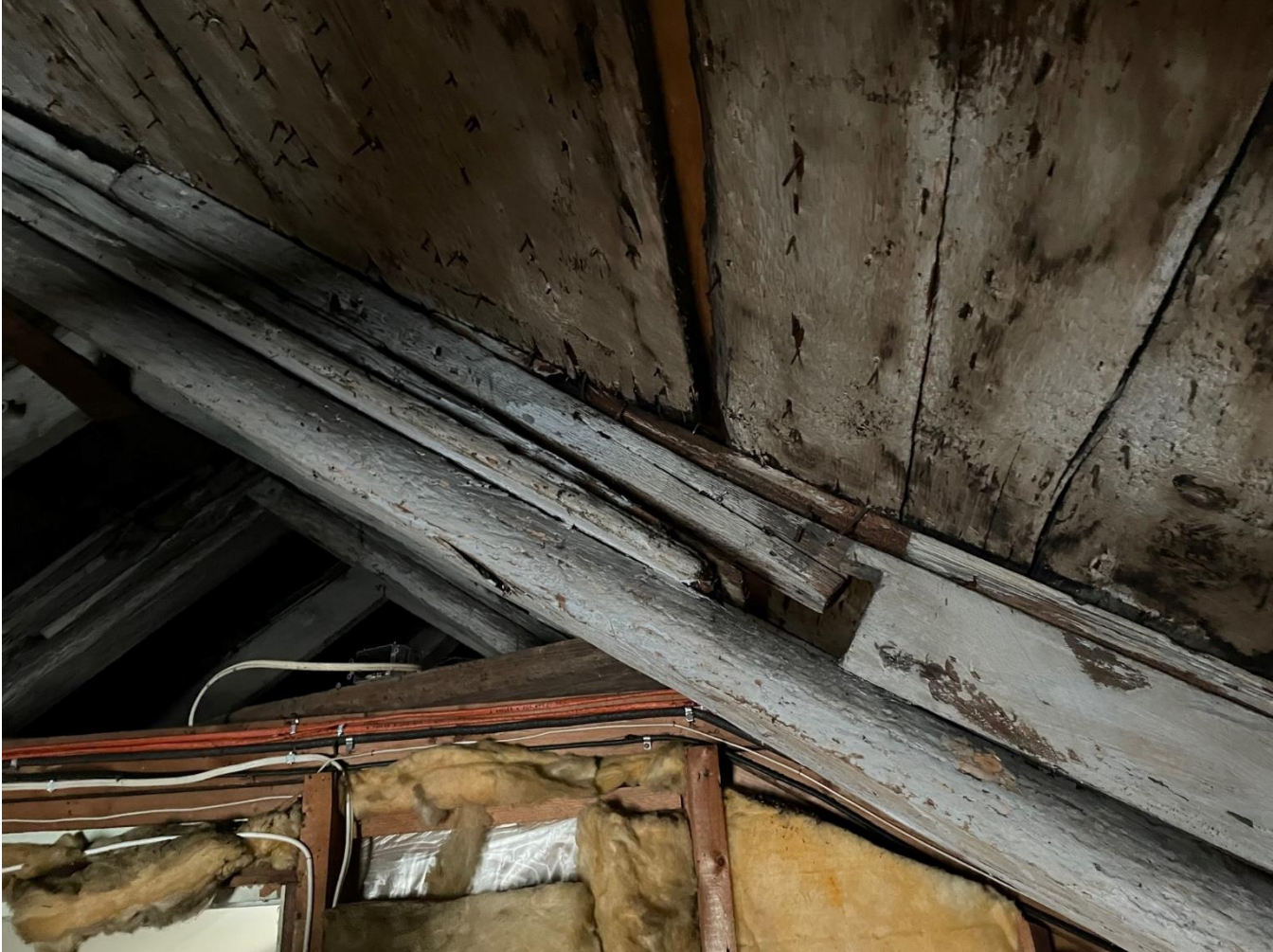
Rafter with shims – March 22, 2022
