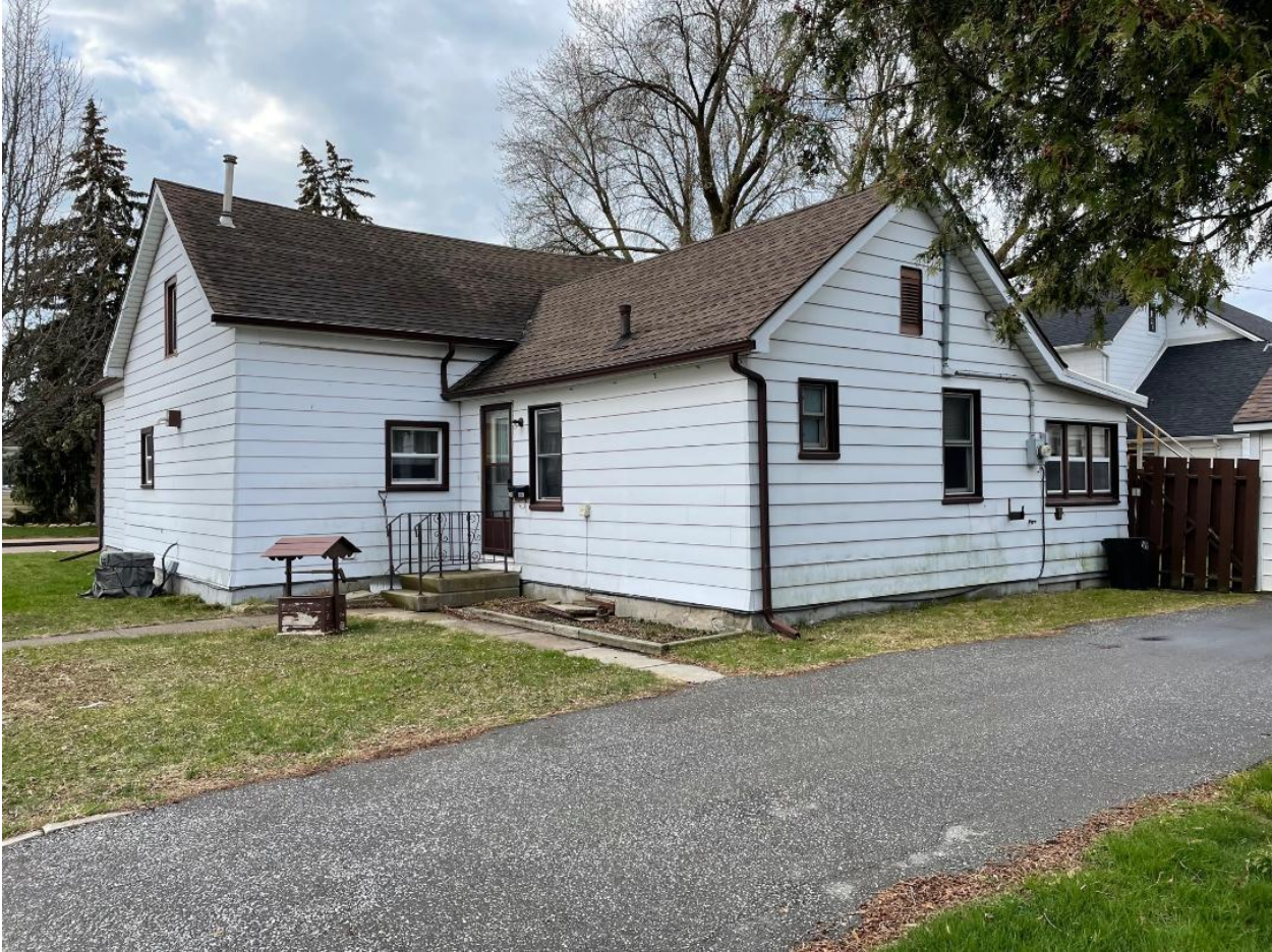
North Façade, Apr. 11, 2022
