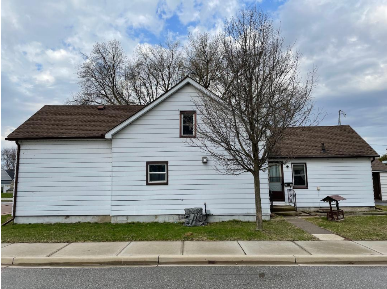
East Façade, Apr. 11, 2022
