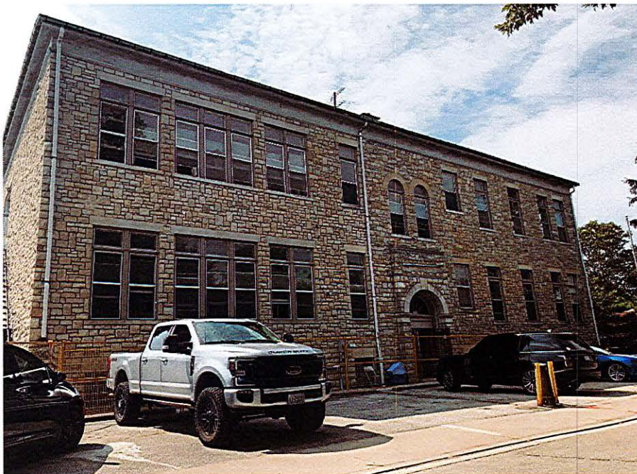
North façade of 247 Brock Street (August 9, 2021)
