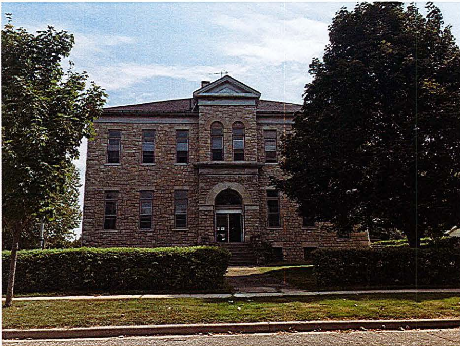
West (Main) façade of 247 Brock Street (August 9, 2021)
