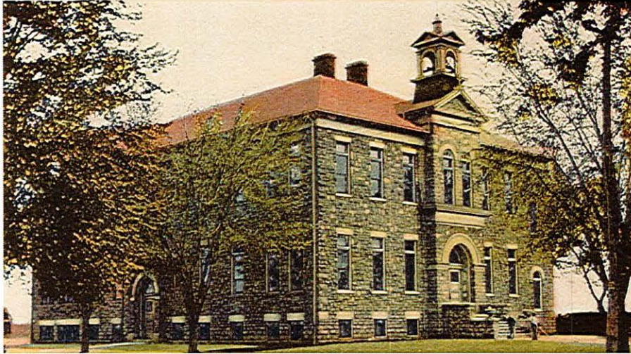
Historic view of West (main) and North Facades, no date, Marsh Collection Society PC100.14
