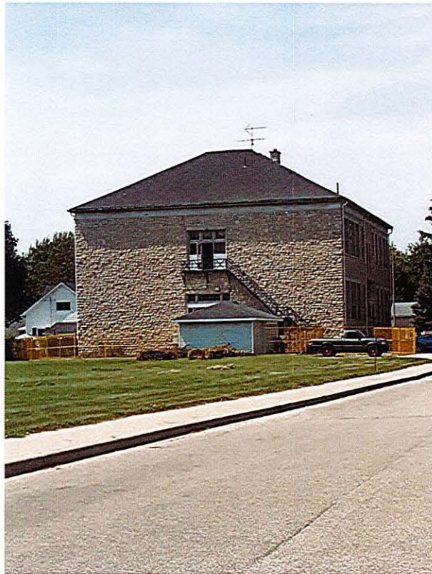
East facades of 247 Brock Street (August 9, 2021)
