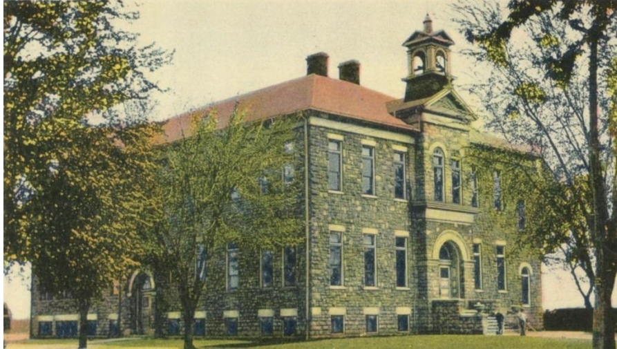
Historic view of West (main) and North Facades, no date, Marsh Collection Society PC100.14
