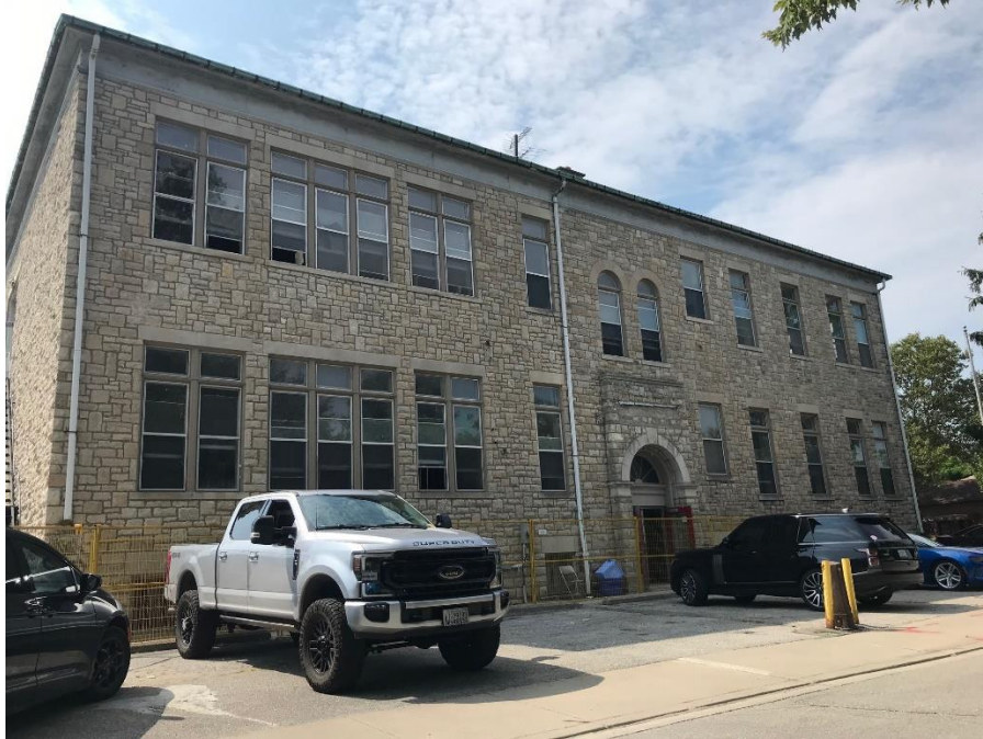
North façade of 247 Brock Street (August 9, 2021)
