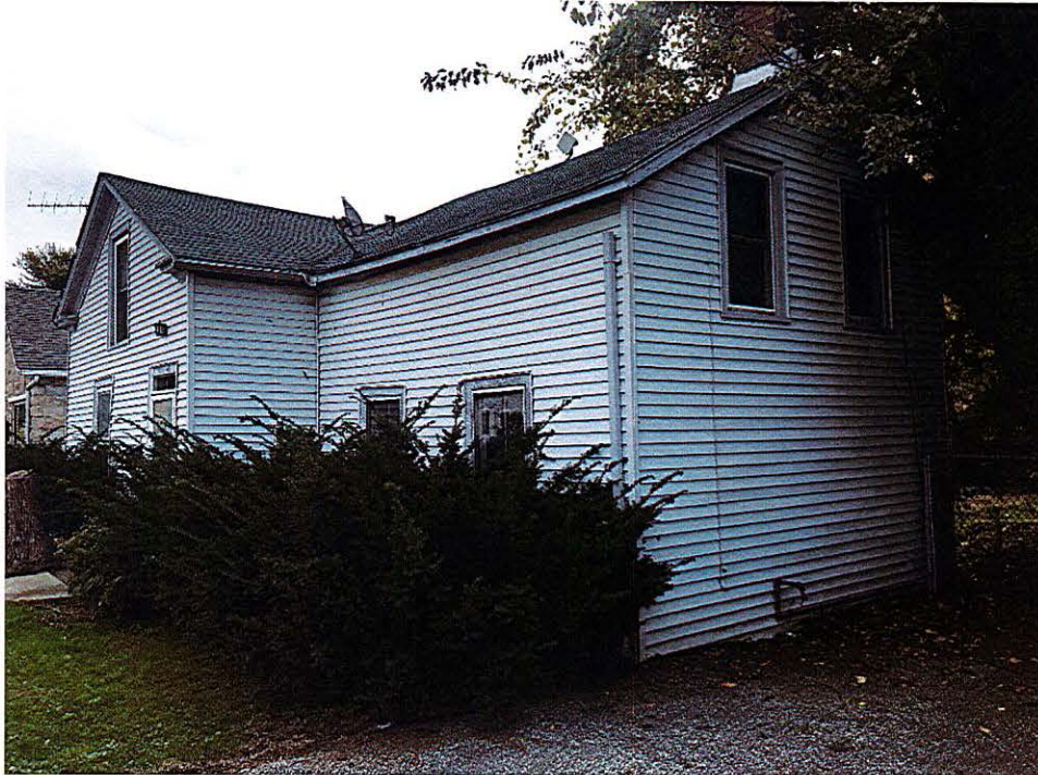
View of west façade, Oct. 7, 2021
