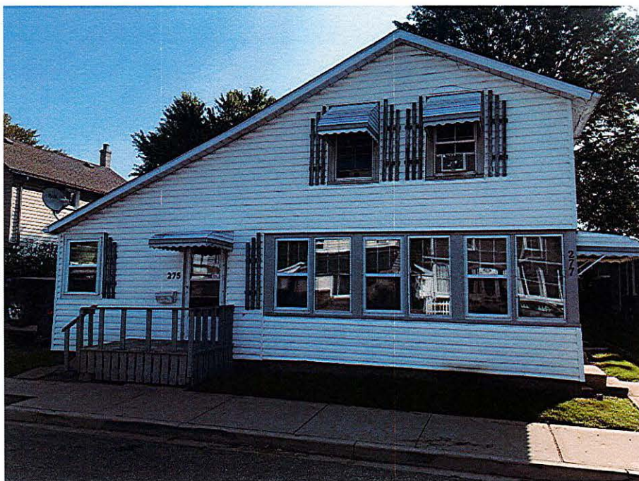
West (Main) façade of 275-77 Bathurst Street (August 27, 2021)
