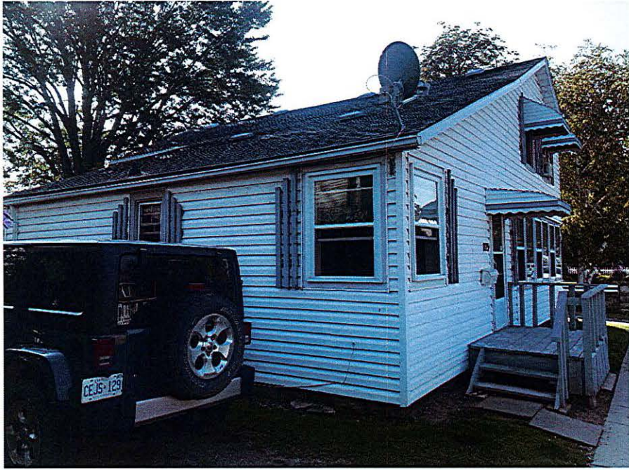
North façade and main (West) façade of 275-77 Bathurst Street (August 20, 2021)
