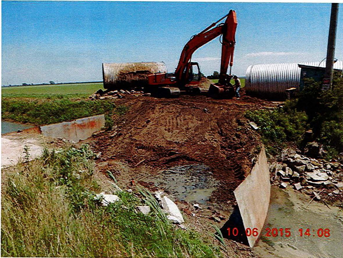
Figure 2. Isolation of Site
