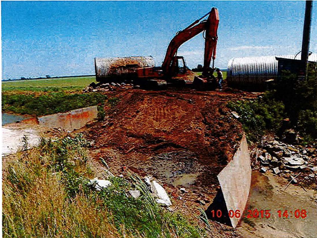
Figure 2. Isolation of Site
