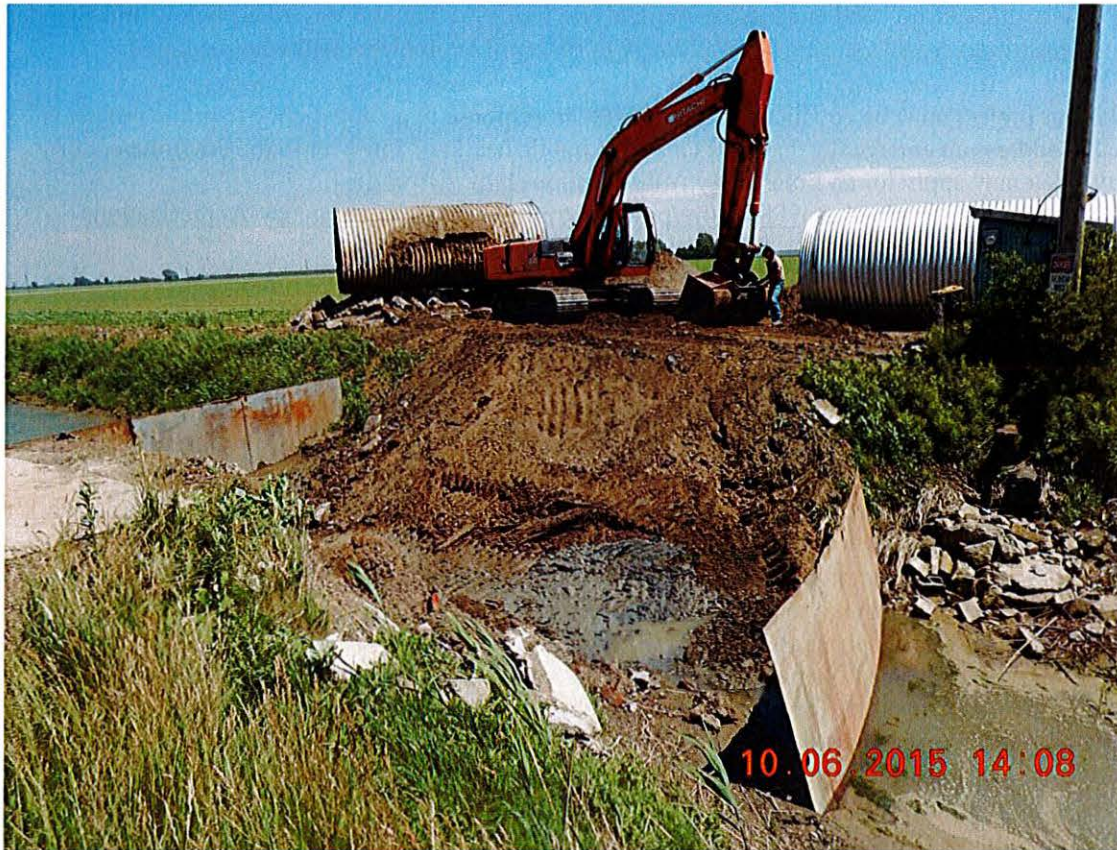
Figure 2. Isolation of Site
