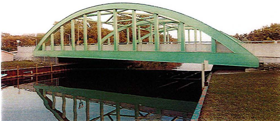
Wyandotte St. Bridge, Completed by FRONT Construction for the City of Windsor, September 2005.
