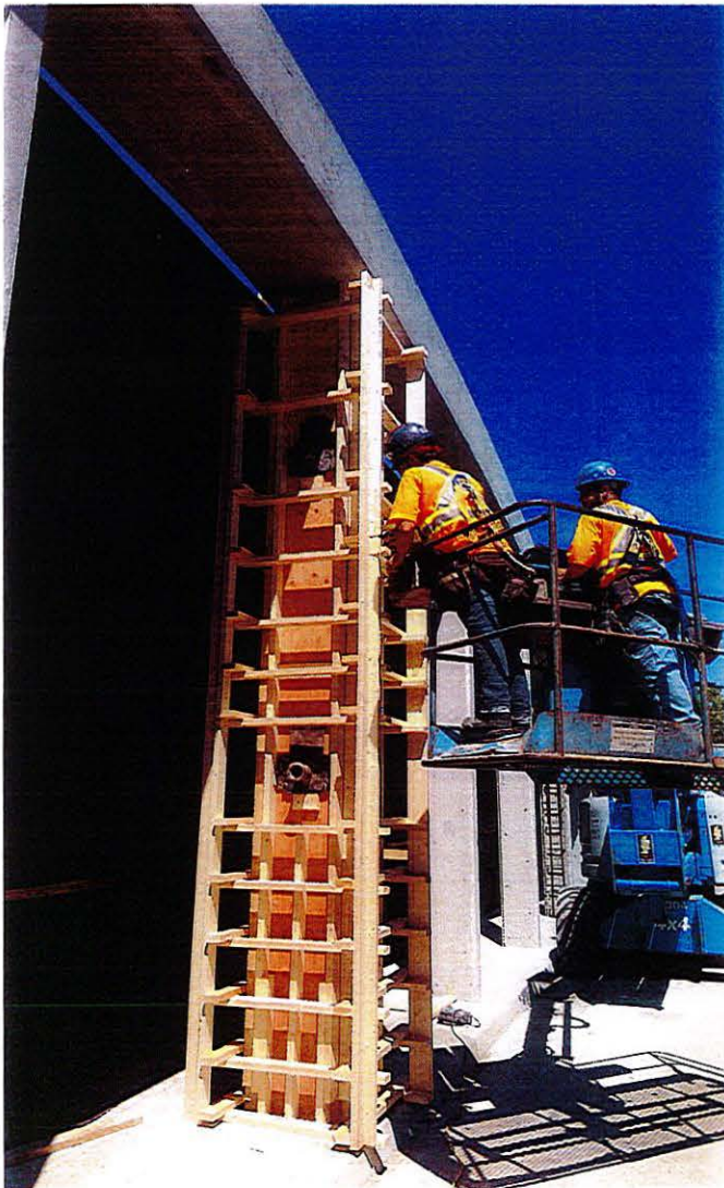
River Canard Bridge Repairs, 2016
