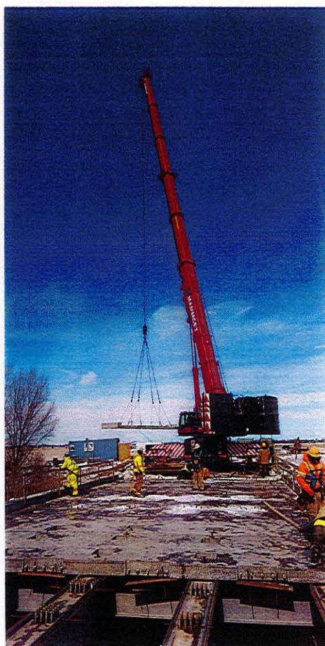
Merlin Rd. Bridge, November 2014
