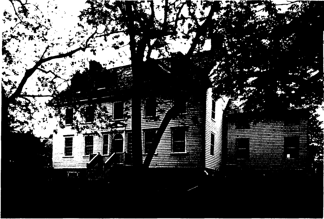
Duff-Baby Historical House - Phase II Exterior and interior restoration. Construct addition with handi-cap lifting device. Windsor, Ontario 1995
