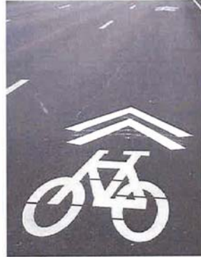
Typical on-road shared cycling/ vehicle lane marking (bicycle symbol with chevrons, or "sharrow")
