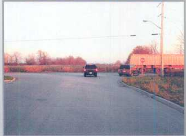
November 22/04, 4:50 pm Jamsyl @ County Rd. #19 looking East
