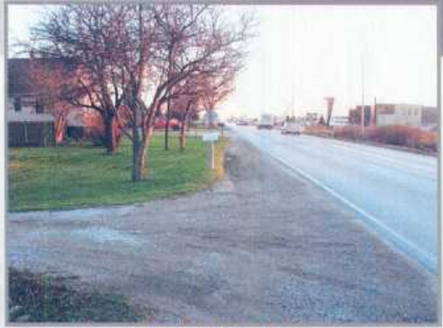
November 22/04, 4:45 pm East side County Rd #19 @ Desro looking south
