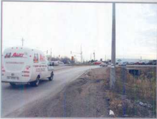
November 22/04, 12:10 pm County Rd. #19 @ County Rd. #22 looking south
