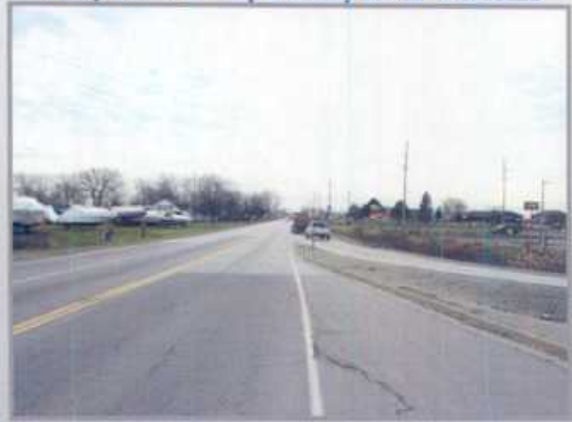
November 22/04, 12:27 pm County Rd. #19 @ County Rd. #22 looking South
