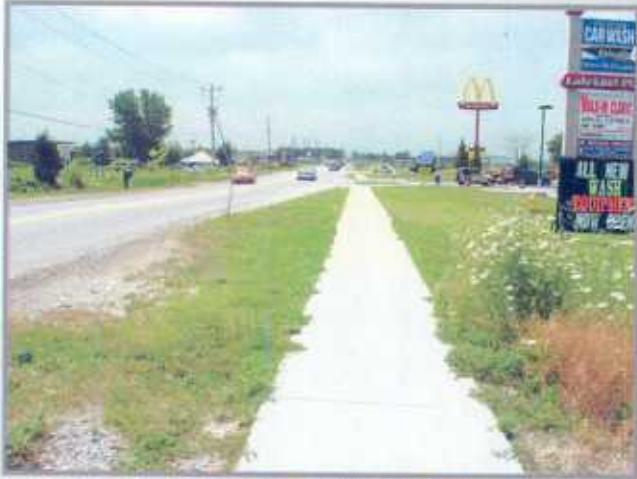
November 22/04, 11:06 am County Rd. #19 @ VIA Rail tracks looking south
